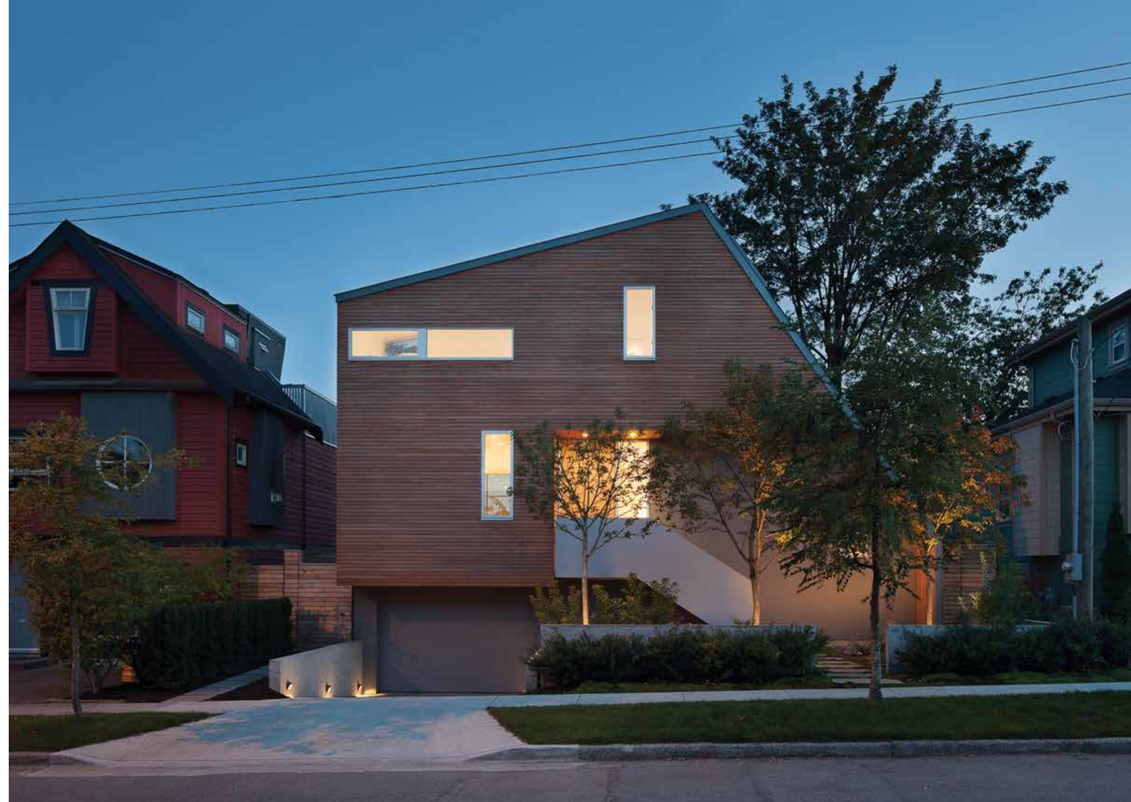
ABOVE East Van House blends West Coast materials, such as cedar slat cladding and a standing-seam metal roof, with clean-lined geometries inspired by Japanese and British minimalism. The resulting house stands out from its eclectic neighbours in the SoMa district of Vancouver.
